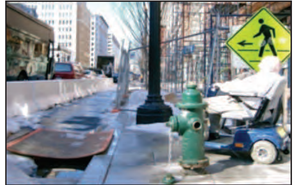
Figure 6. All Ramps Should be Firm, Stable, and Have a Non-Slip Surface
