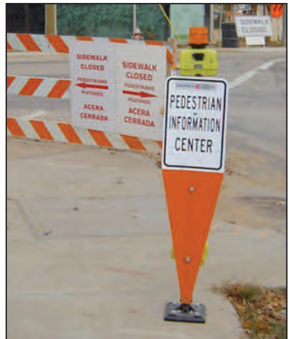
Figure 4. Audible Information Device in Advance of a Closed Sidewalk
